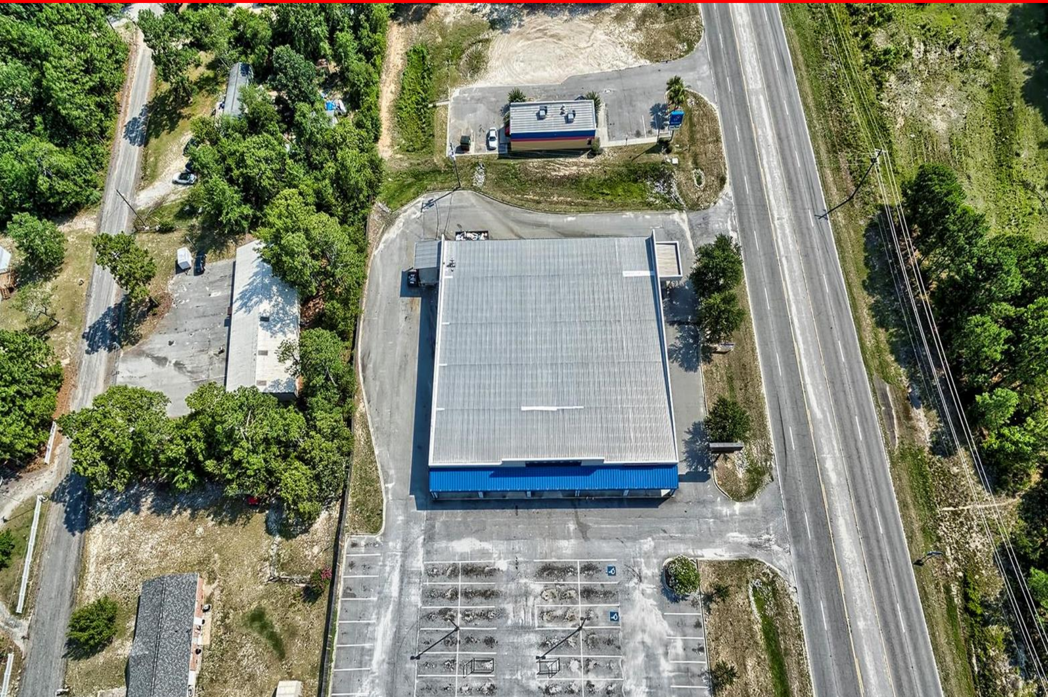
Former Fred's Pharmacy multiple points of ingress and egress and a large parking lot
